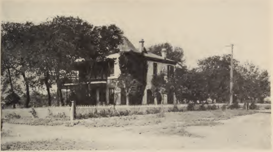
THE PROPOSED SITE OF THE NEW SAINT PHILIP'S
